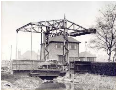
The old Meccano Bridge West Bridgford
