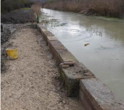
Bob eyes up the pilings at Lock 14 upper landing which was completed in December and Dave, Mark, Tony K & Martin build up the copings in bitterly cold weather early January.
