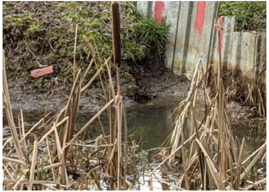
Above: Leak at culvert 39 Below: Leak at culvert 42
