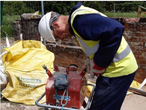
Inevitable brick cleaning - not as easy as it may look when in the hands of professionals!
