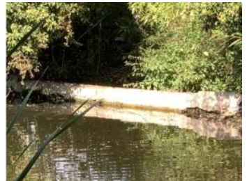
Very Low Level at Overflow Weir
