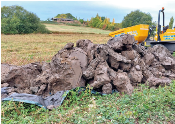
That's a lot of puddle clay! and (right) the clay being compacted into a trench to prevent water ingress
