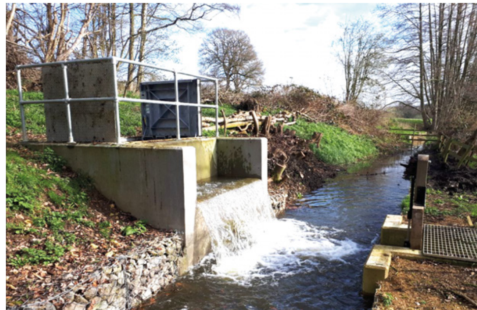
Clearance work on the Knipton feeder showing good results
