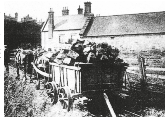
Next to the Peacock Inn, where a second horse would be added for the steepest part of the climb - note the trailing sprag on the waggon.
