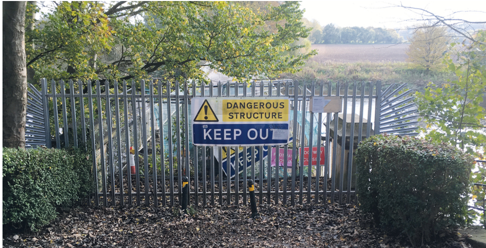
Old Tram Bridge carrying the tramroad linking the two sections of the Lancaster Canal across the River Ribble in Preston.
